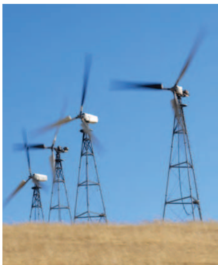
First-generation turbines have latticed towers that attract some raptors.
